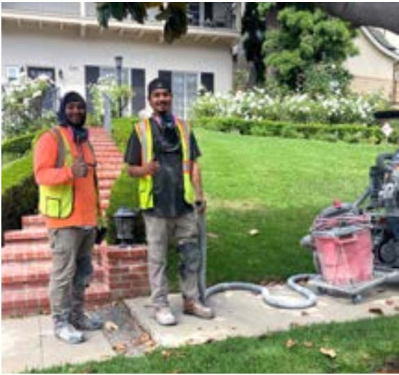
Crew from Precision Grinding take on sidewalk safety measures
